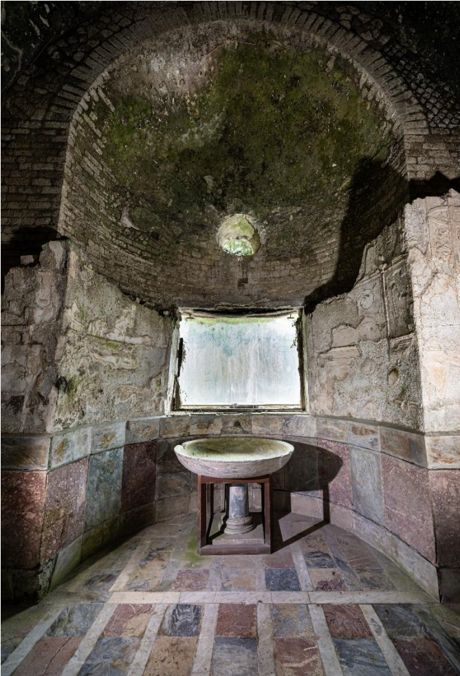
Calidarium before restoration
