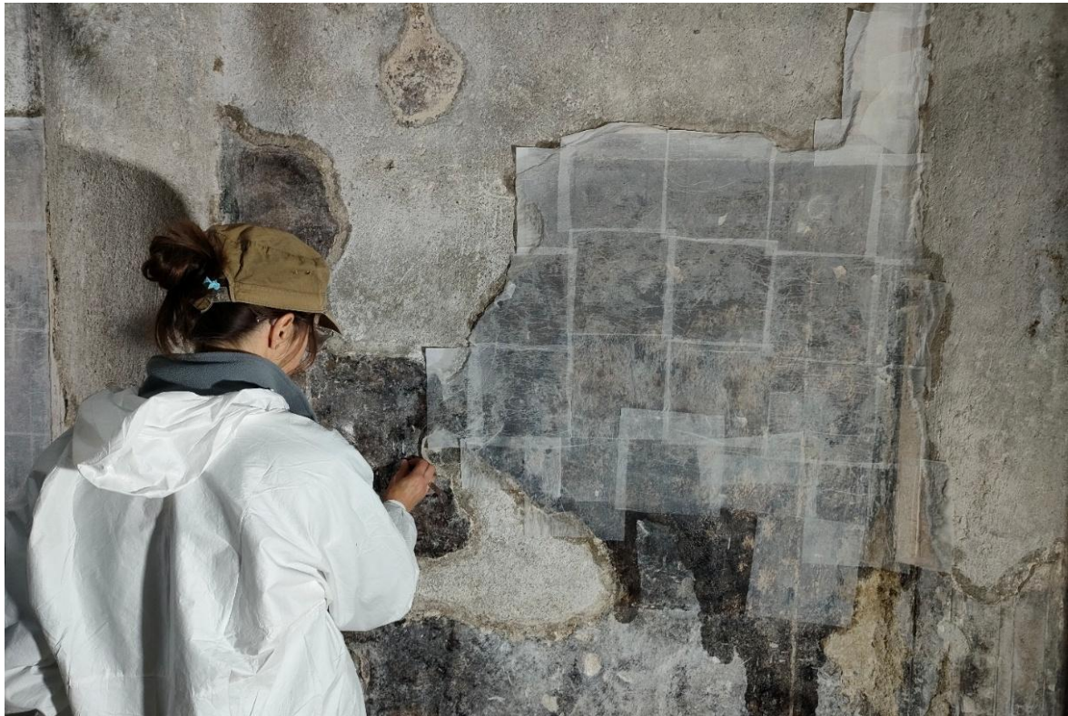
Cleaning works on the frescoed wall of the belvedere hall
