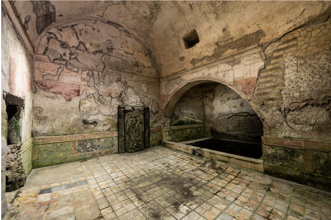
Frigidarium before restoration
